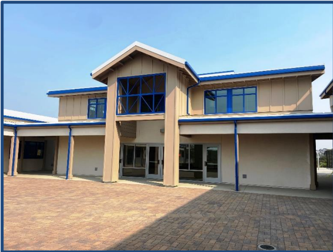
Sunset High School / Campus Re-construction
