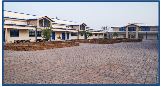
Sunset High School / Campus Re-construction
